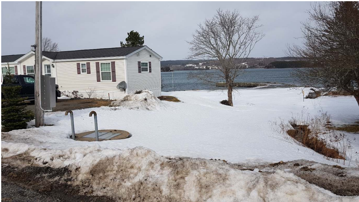
Figure 5-11: (2) Marine Drive near North Street Sewage Lift Station – Guysborough
