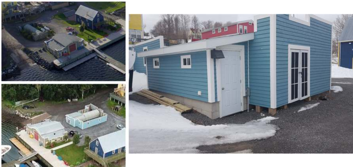
Figure 5-2 Main Street Rotating Biological Contactor - Guysborough
