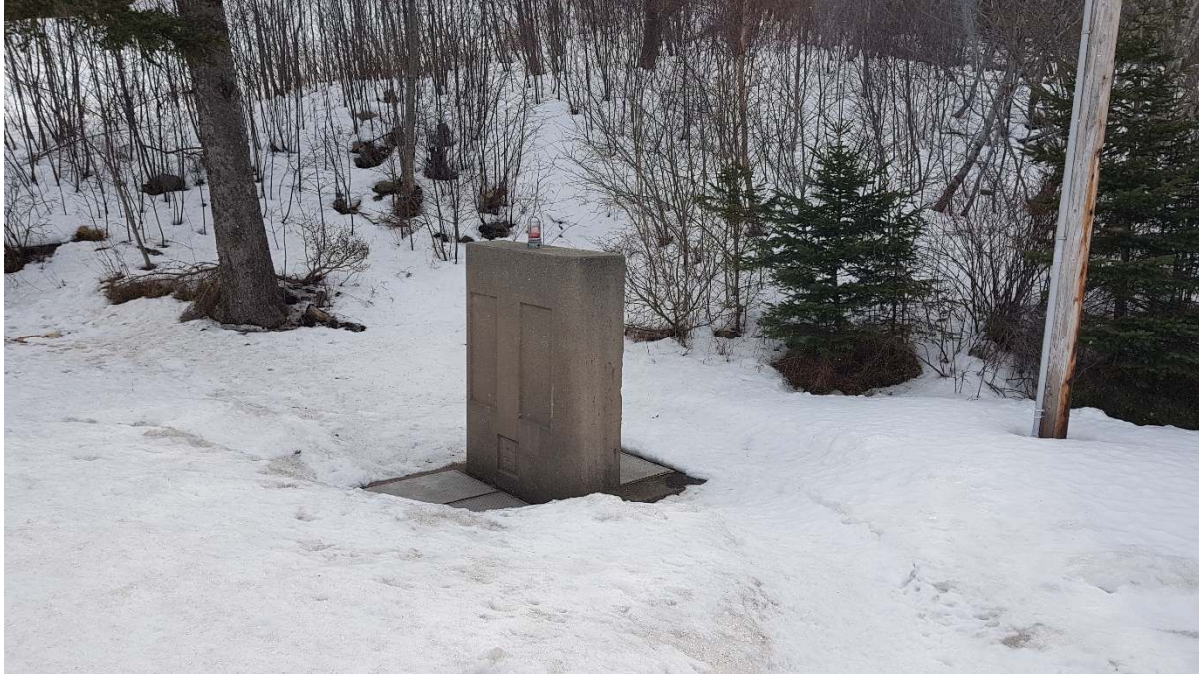
Figure 5-10: (1) Marine Drive Sewage Lift Station - Guysborough
