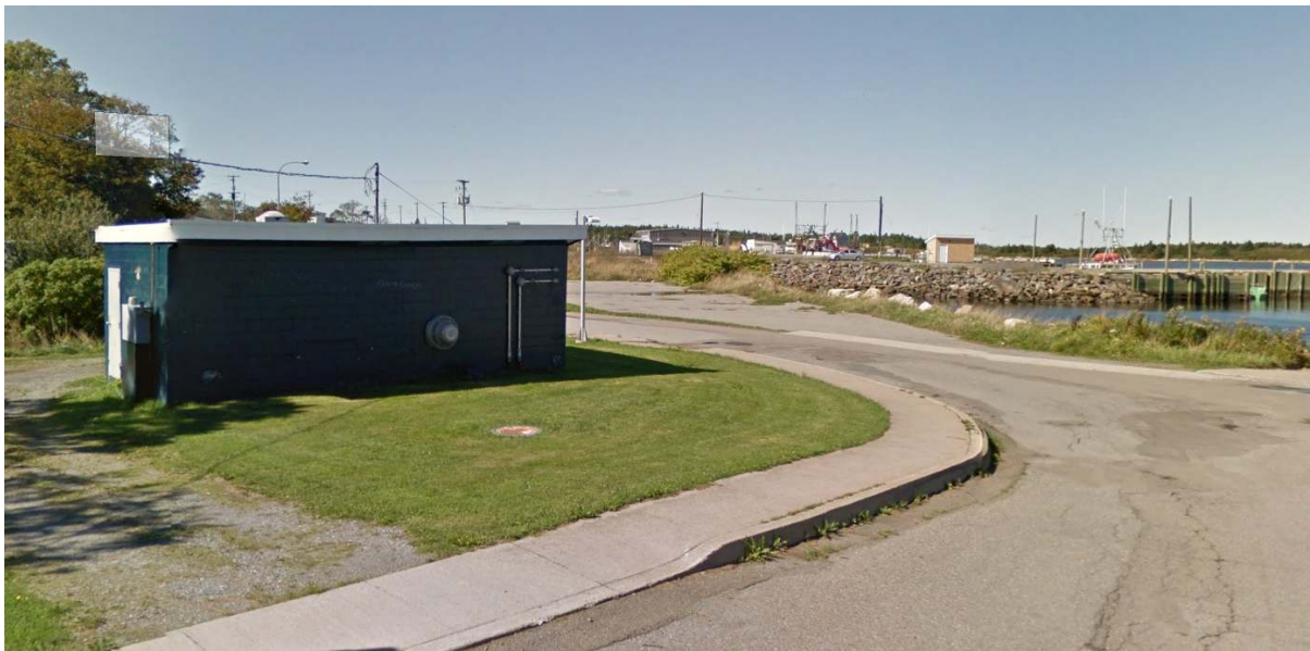
Figure 5-16 (7) Water Street Sewer Lift Station - Canso
