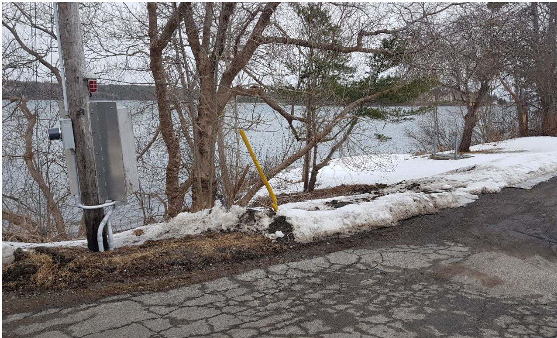
Figure 5-12: (3) Main Street near Russell Lane Sewage Lift Station – Guysborough
