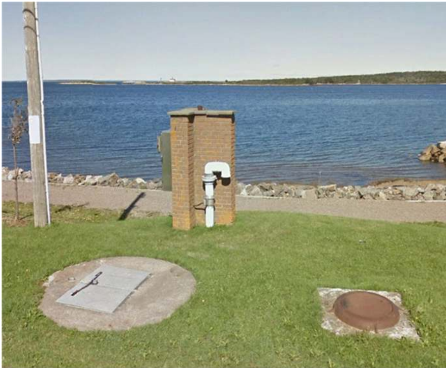
Figure 5-17: (8) Union Street Sewage Lift Station - Canso
