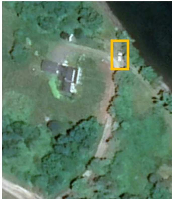
Figure 5-14: (5) Lower Water Street Sewage Lift Station – Guysborough
