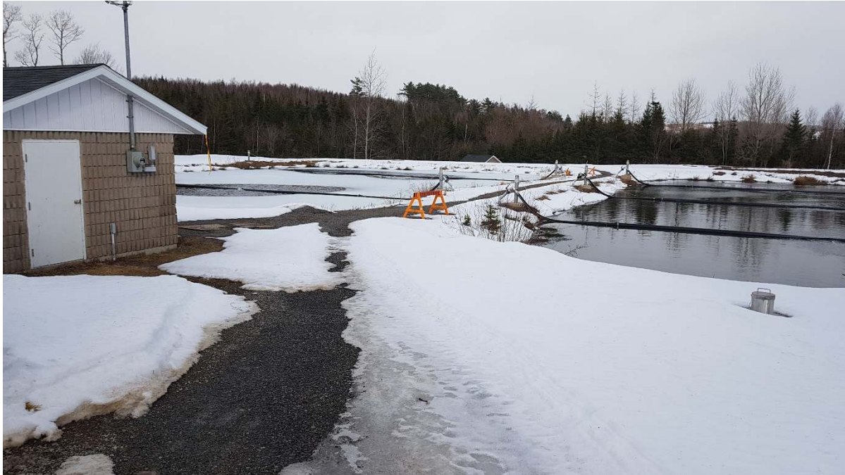
Figure 5-3: Wastewater Treatment Lagoon - Guysborough
