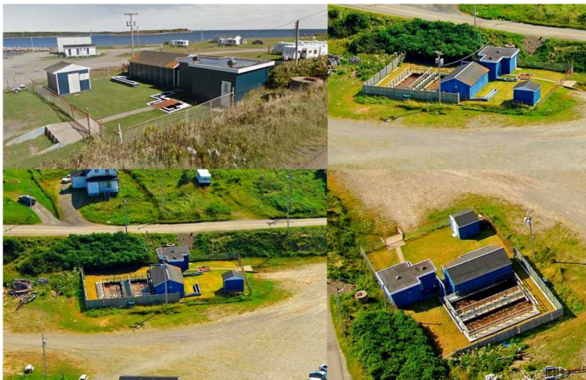
Figure 5-5 Union Street Activated Sludge Plant - Canso
