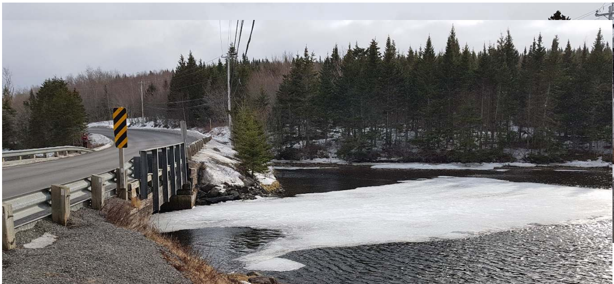
Figure 5-19: Coastal Water Level proximity in reference to road and bridge elevations in the Municipality of the District of Guysborough
