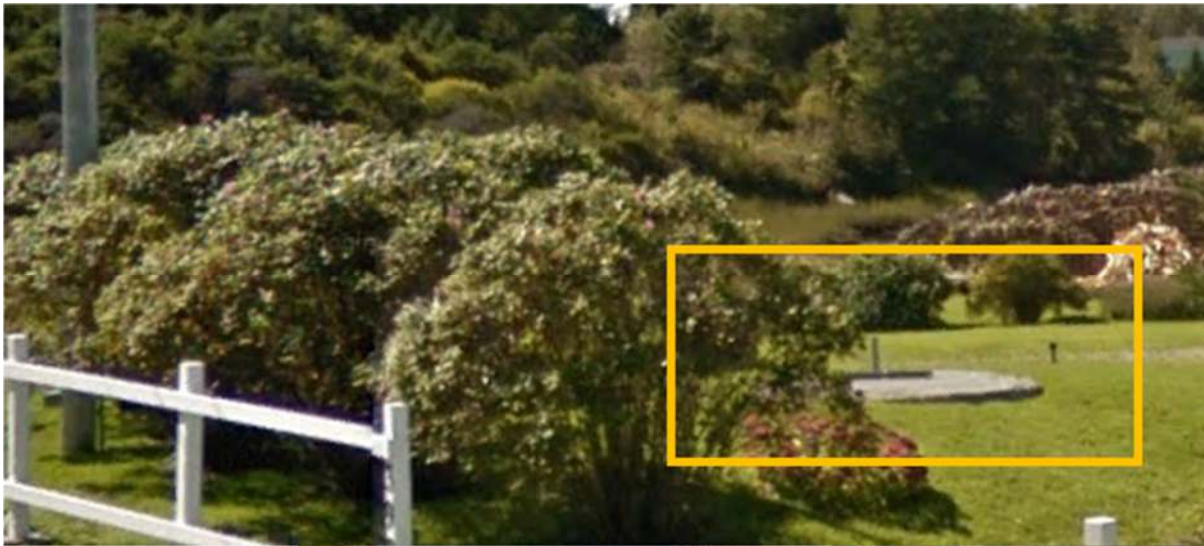
Figure 5-15: (6) End of Water Street Sewage Lift Station – Canso
